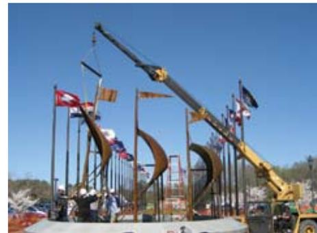
Sections of the sculpture were transported to Jamestown Settlement by truck from Virginia’s Eastern Shore, lifted into place with a crane, and secured to the Quadricentennial Plaza fountain with a stainless steel base anchoring system.
