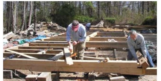
Jamestown Settlement exhibits fabrication staff are building sections of the row house frame in a service area before erecting the frame on the building’s cobblestone foundation.
